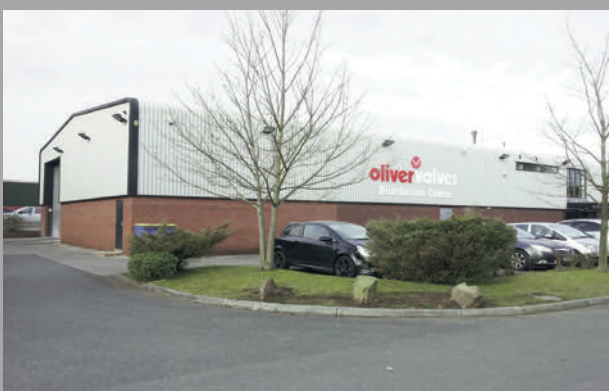
Oliver Distribution Centre
