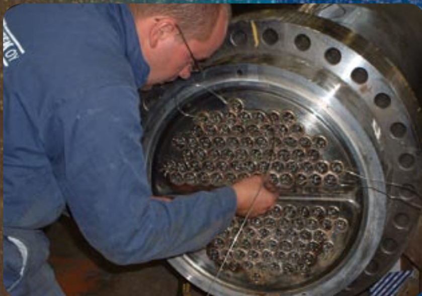
hiTRAN installation. Courtesy: KCC
